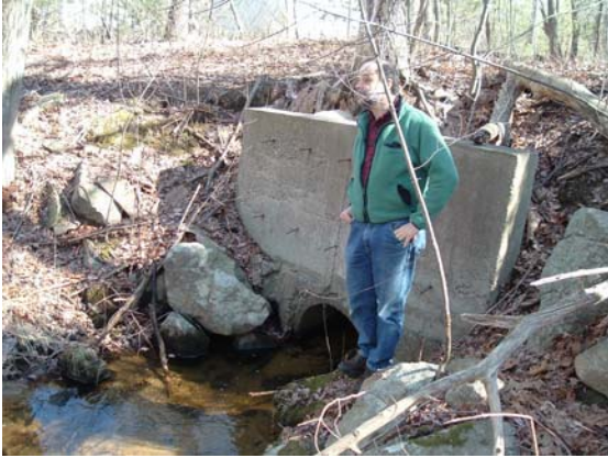
Larry Soucie checking culverts for sediment
